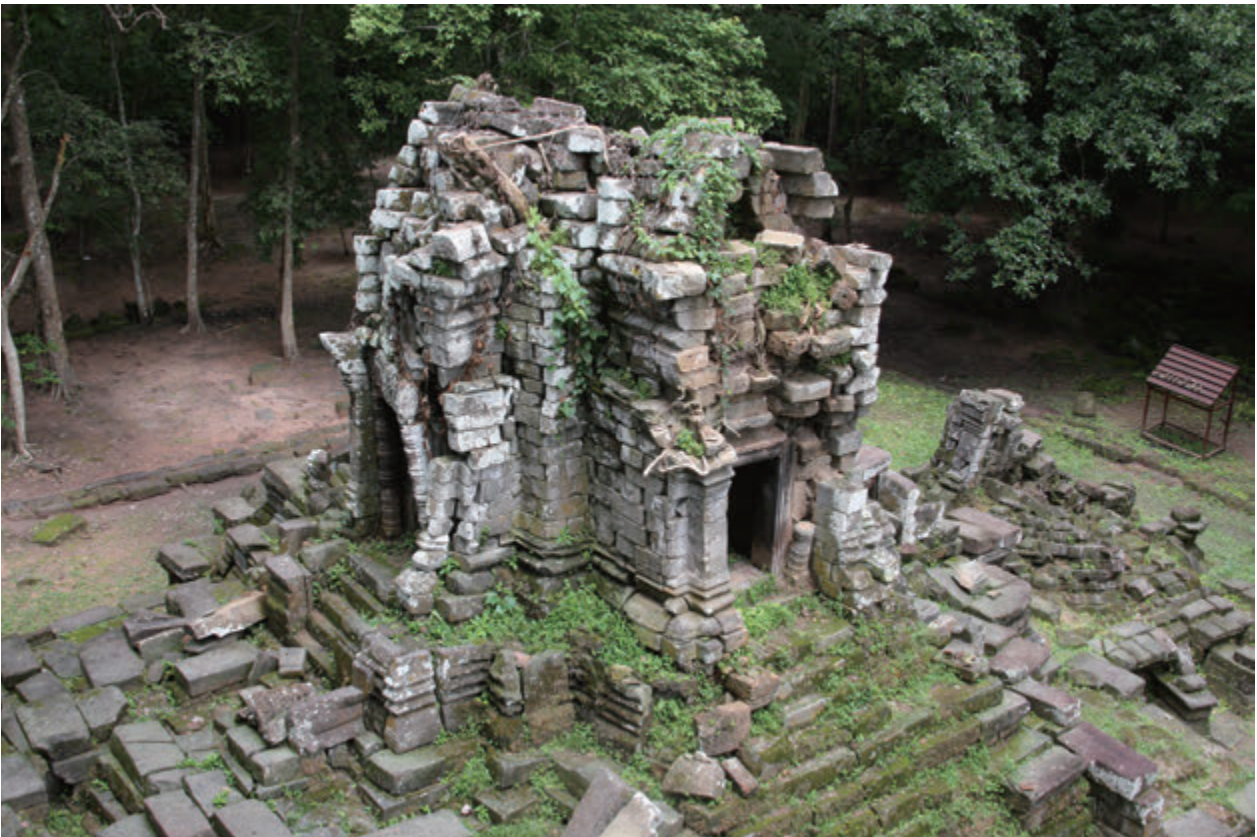
Fig. 6 Central sanctuary before reconstruction (view from the southeast)
