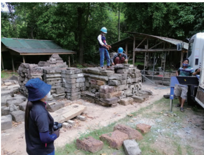
Fig. 12 Trial reassembly of the upper part of the building frame
