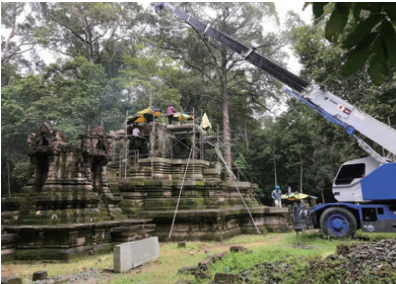
Fig. 8 Reconstruction situation of Central sanctuary (view from the northwest)
