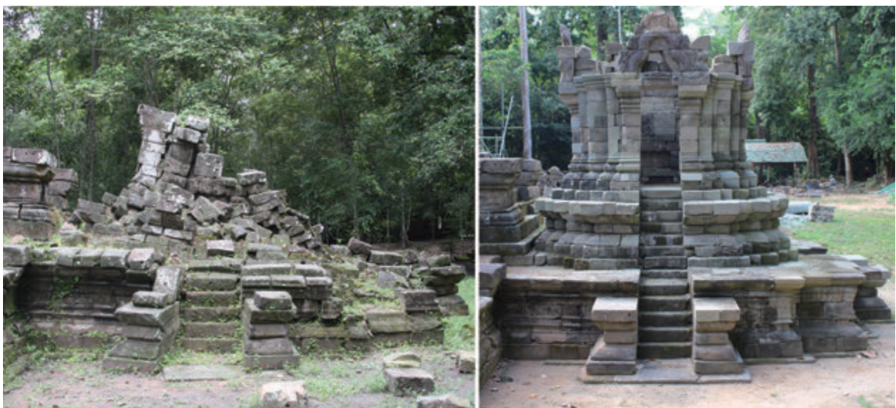
Fig. 3 North sanctuary before the reconstruction (left side), after the reconstruction(right side) (view from the east)
