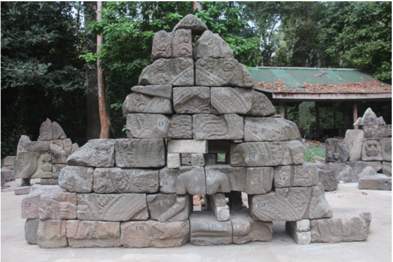
Fig. 13 Trial reassembly of the first east pediment
