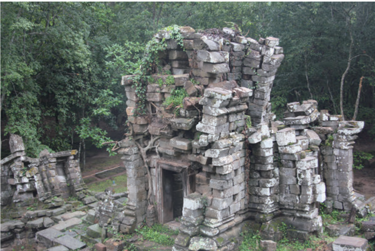
Fig. 11 Central sanctuary before dismantlement (view from the northeast)
