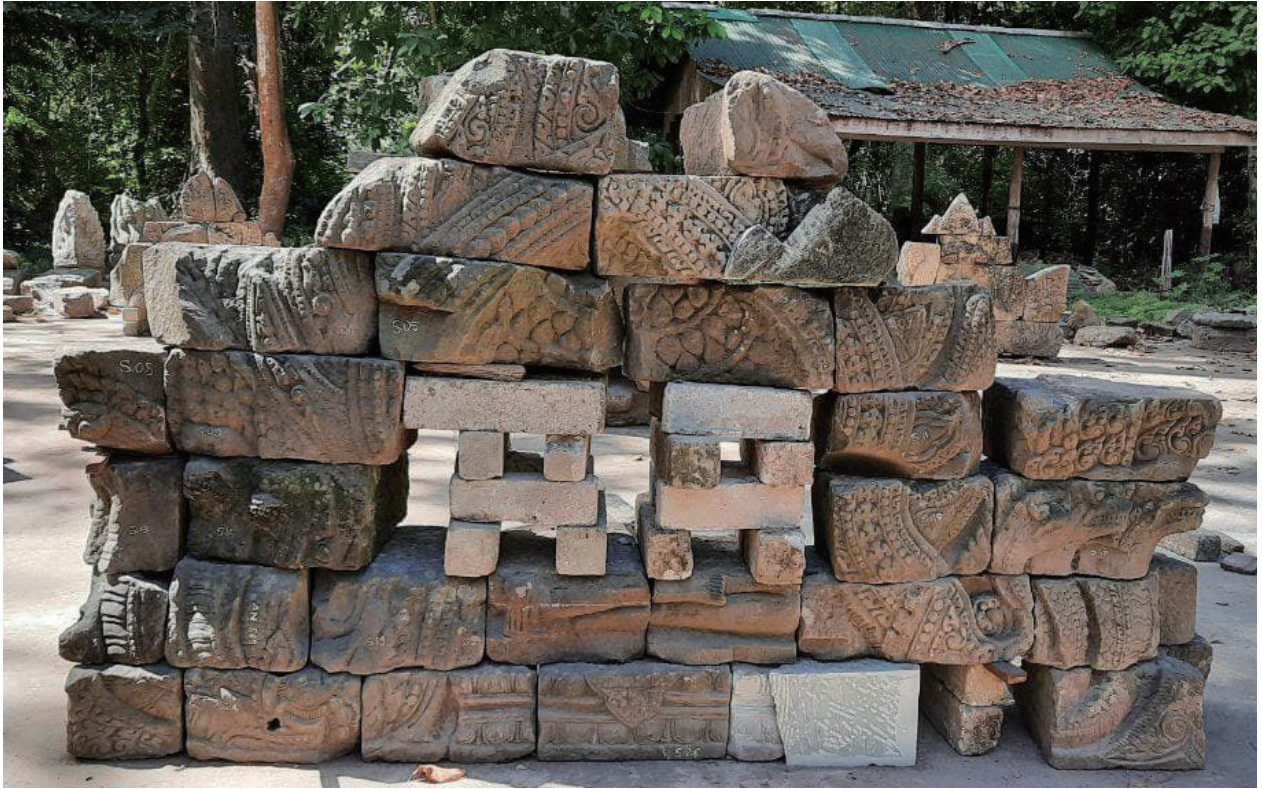
Fig. 15 Trial reassembly of the first south pediment
