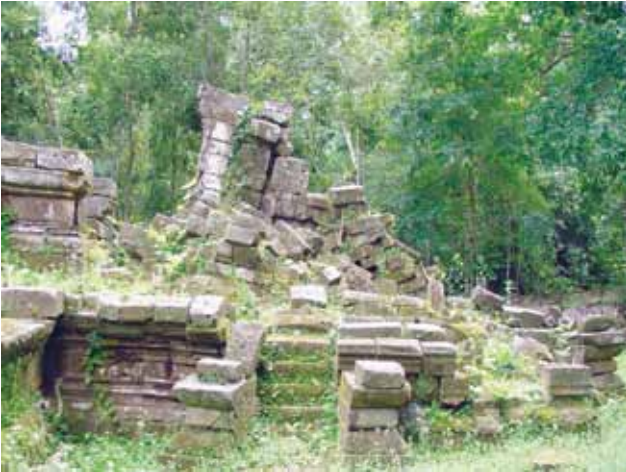
崩壊の著しい北祠堂 Notably crumbling North Tower
