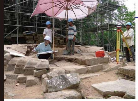
南祠堂の建物解体後、その基壇の不同沈下の度合いを測量機器で計測する Measuring the degree of differential settlement of the foundation by surveying instrument after the dismantlement of upper building of the Southern Sanctuary
