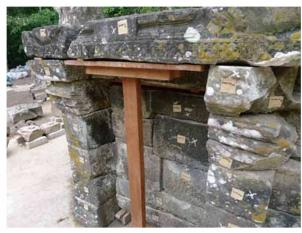
解体された建物の各部材にはマーキングが施されており、本来の位置に復元することが可能となる Each stone member of the building is marked according to its position, in order to reassemble the building as its original form
