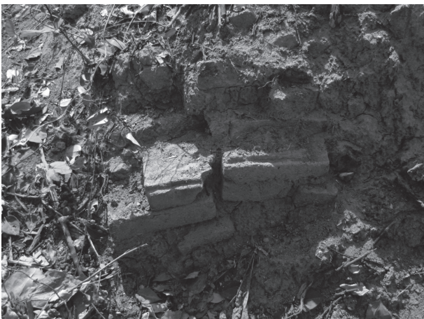
Fig.50 Brick remains No. 1
