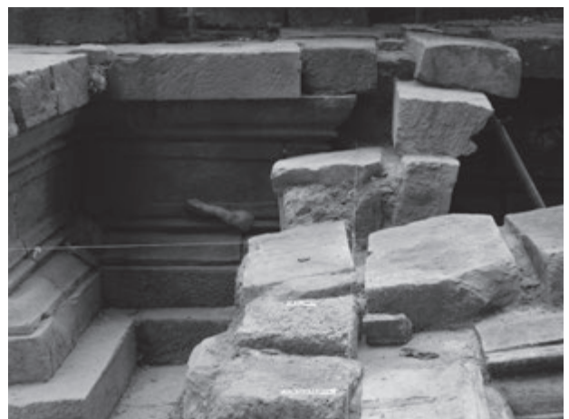
Fig. 11: Connecting area with the Central Sanctuary (view of east side)
