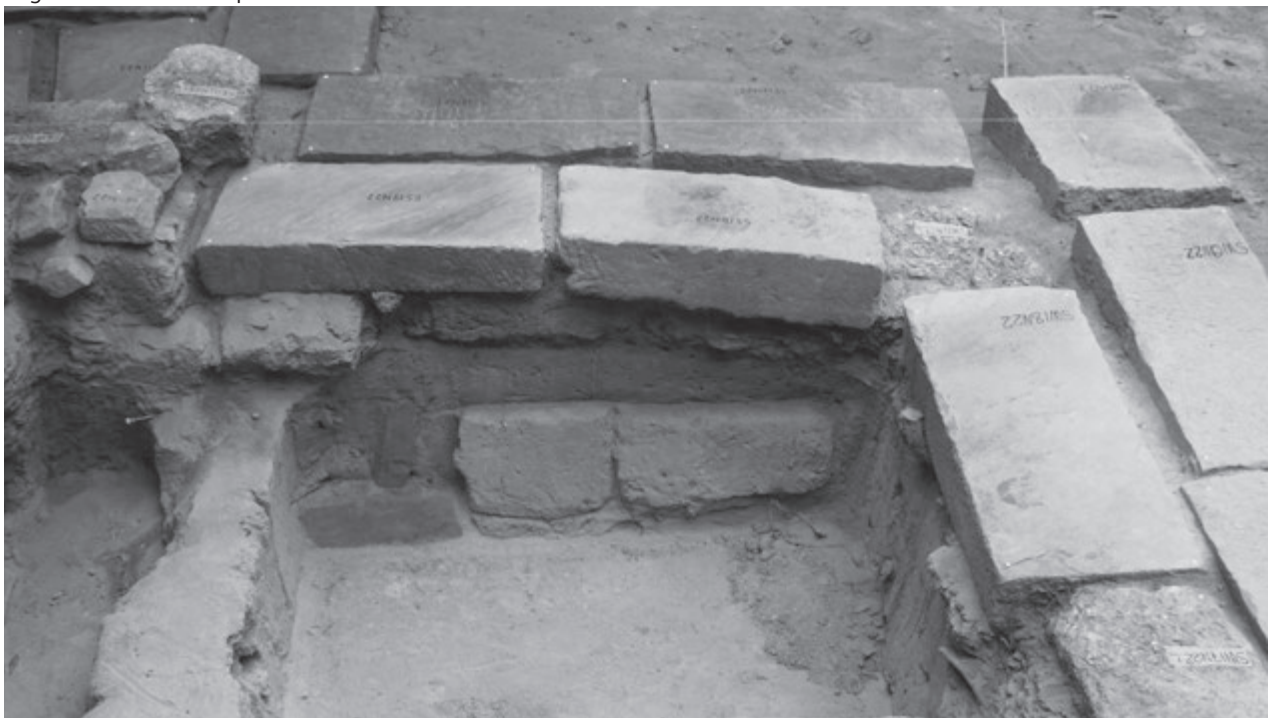
Fig. 21: Relationship between the stone blocks on the south side of N22, stone blocks of N23-N25 and the east-west stone line in the foundation
