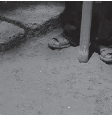
Photo 16: Leveling and compacting using a round rammer
