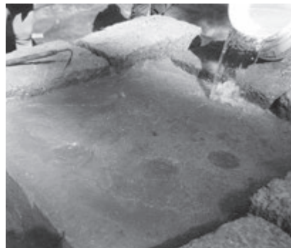
Photo 26: Water supply test after curing
