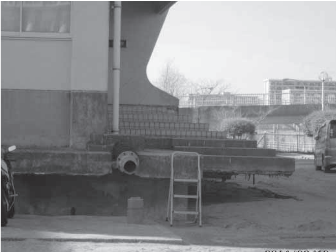
Photo 7: Ground subsidence caused by liquefaction in Urayasu in the wake of the Great East Japan Earthquake
