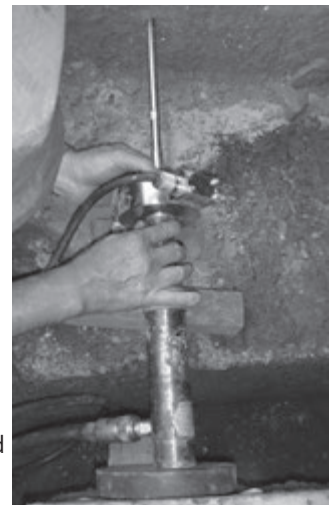
Photo 27: Confirmation of erosion resistance and inspection of the side walls after curing
