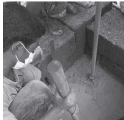
Photo 17: Compacting using an "elephant's foot" rammer
