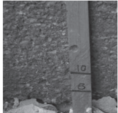
Photo 15: Soil spreading thickness and compacted thickness
