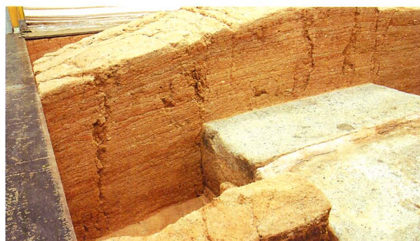
石室に沿って版築を突き破る地割れ Fissures following the stone chamber, splitting layers of tamped earth
