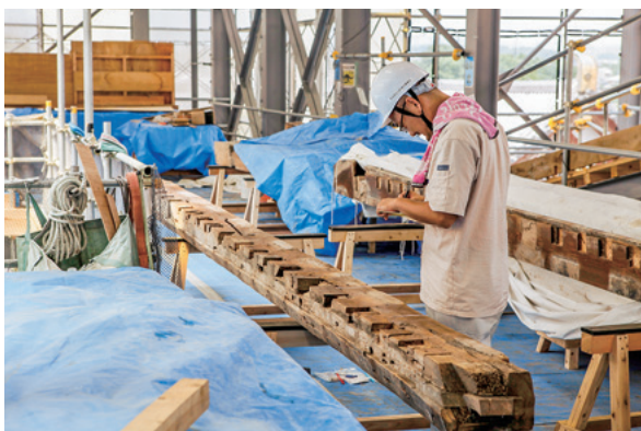
年代学研究室：薬師寺東塔解体修理にともなう年輪年代調査 Dendrochronological Dating Section: Dendrochronological investigation in conjunction with the dismantling and repair of the Eastern Pagoda, Yakushiji temple
