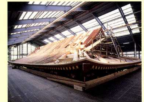
Building up rafters and constructing roof
