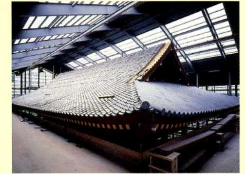
Covering with roof tiles
