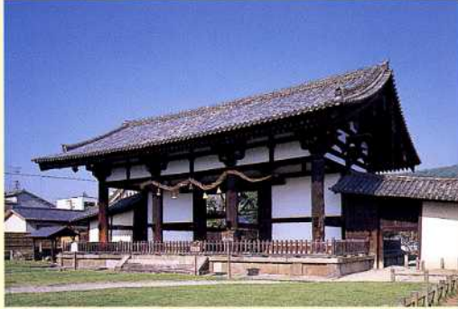
Tegai Gate of Todaiji temple (erected in the middle eighth century) (Referred to for the size and proportions of the separate components, as an example of large building in the Nara period)
