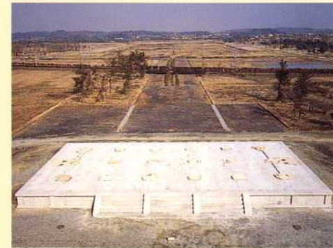
Reconstruction of platform
