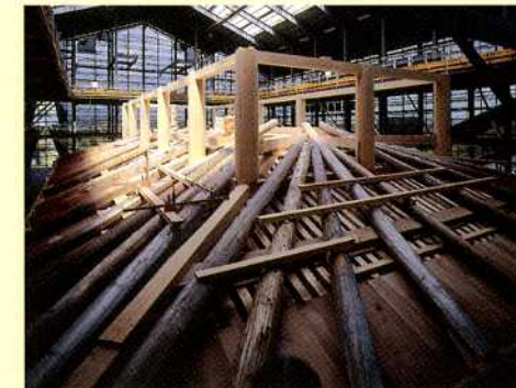
Building the second story
