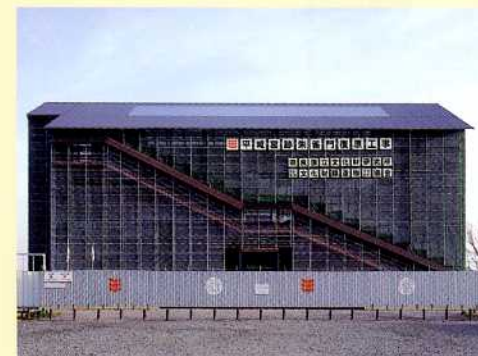
Construction of shelter building (For scaffolding and weather protection)
