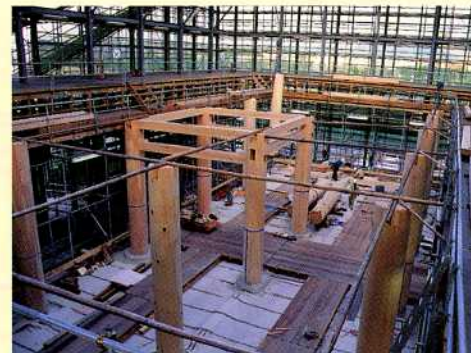
Erecting pillars and jointing them by pillar-top brace
