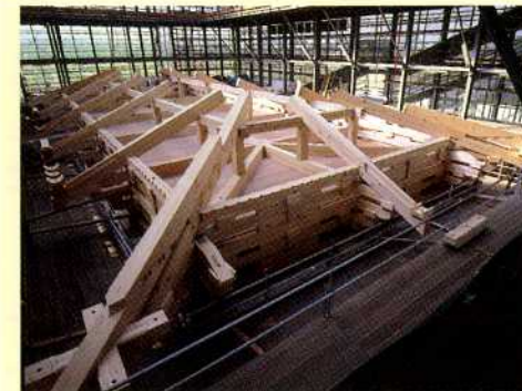
Completion of building of the first story
