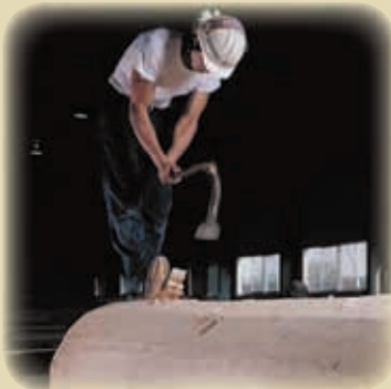
Shaping and finishing of architectural members was done with ancient tools. In addition to shaping with a planing tool ( yariganna , left), pillars are worked with an adze-like chōna .
