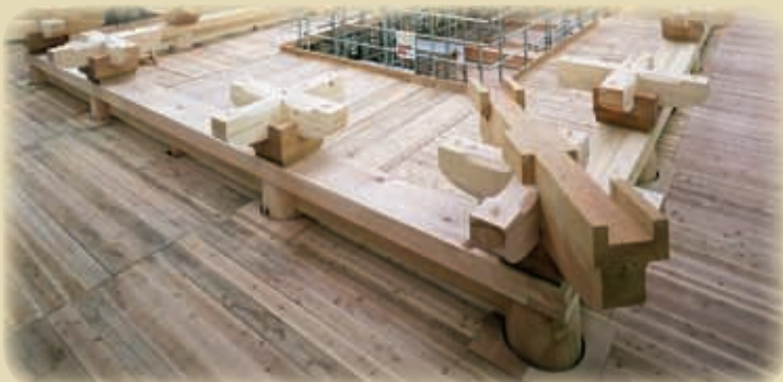
Japanese cypress was used for most of the members. For the principal bearing blocks of bracket complexes and other parts where load concentrates, the ancient practice of using zelkova was followed.
