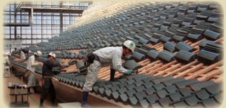
In order to reduce the load of the roof, no layer of soil was used in laying the tiles, which were attached individually to the laths with copper wire.
