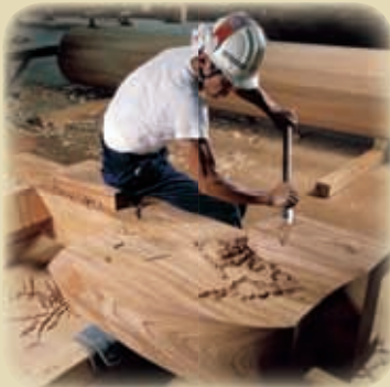
Shaping and finishing of architectural members was done with ancient tools. In addition to shaping with a planing tool ( yariganna , left), pillars are worked with an adze-like chōna .
