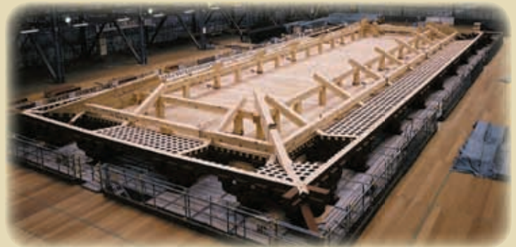
Characteristics of ancient architecture are utilized not only in the external appearance, but also in the structure. While seismic dampers were employed, it was possible to minimize other reinforcement.
