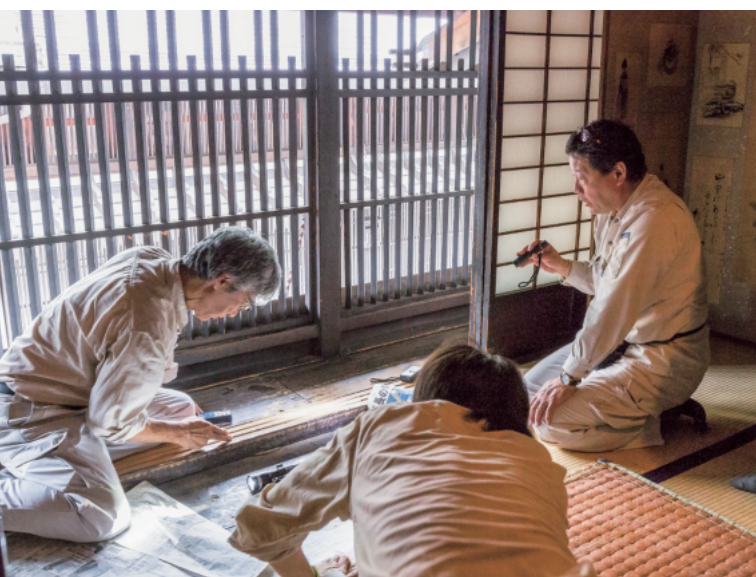
建造物研究室：旧中村家住宅（長野県塩尻市）の調査 Architectural History Section: Investigation of the Former Nakamura Residence (Shiojiri, Nagano prefecture)
