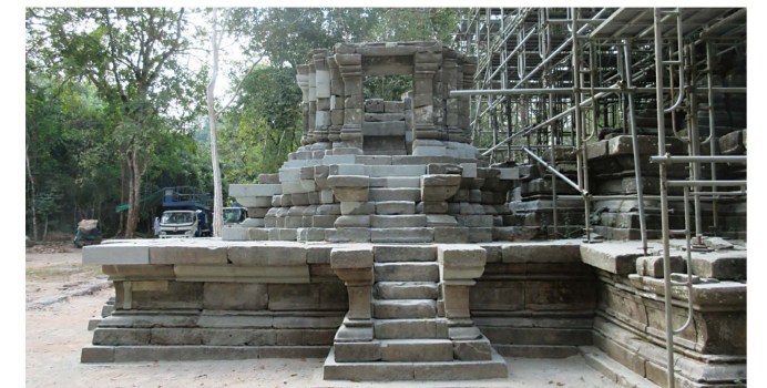
Southern Sanctuary: Before restoration (above), After restoration (below)
