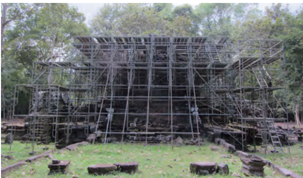
Fig. 2 View of scaffoldings (view from the east)
