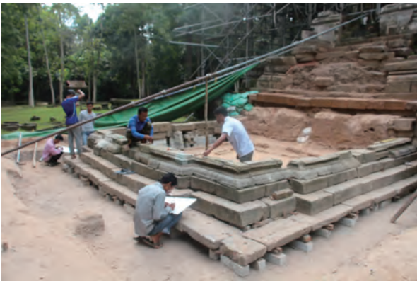
Fig. 14 Reassembly of the northern sanctuary
