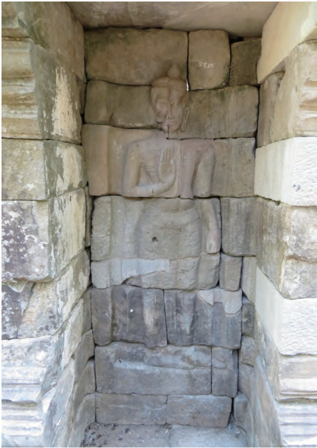
Fig. 17 Reassembled south false door of the northern sanctuary (view from the south)
