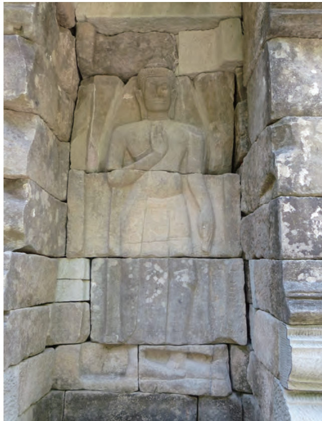
Fig. 16 Reassembled west false door of the northern sanctuary (view from the west)
